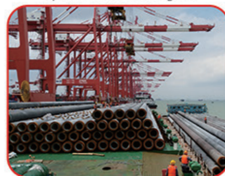
70米超长管桩集港 70m Spun Pile Congregation
