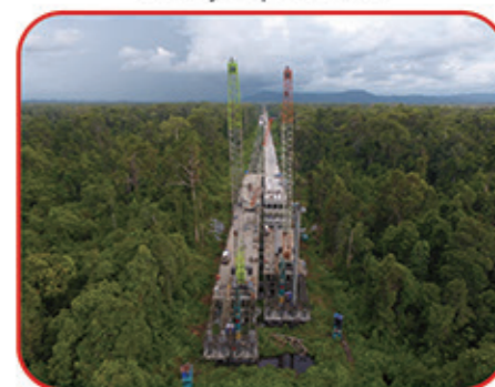
淤泥沼泽地吊锤法施工 Drop-Hammer Construction Method in Mud Swamp
