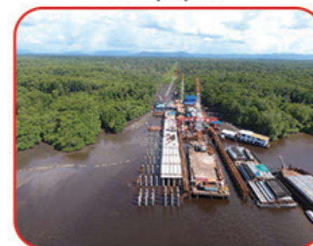
浅滩区域施工 Construction in Shoal Area
